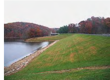
Tom Jenkins Dam and a
